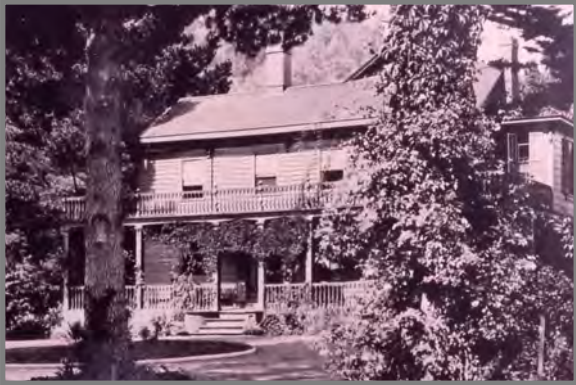
The "Sunnyside" home built by the Worns in the 1880s
